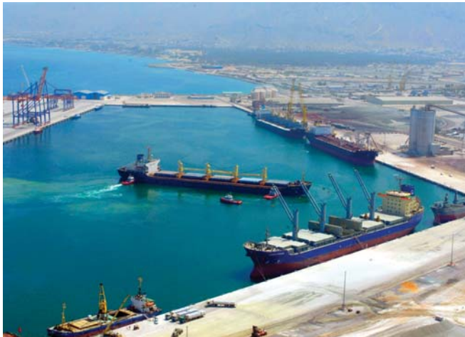
Vessels are loaded and unloaded the same day at Saqr Port.
