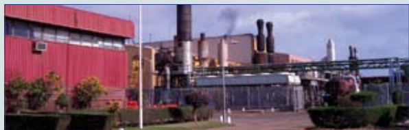
Kotu Power Station
