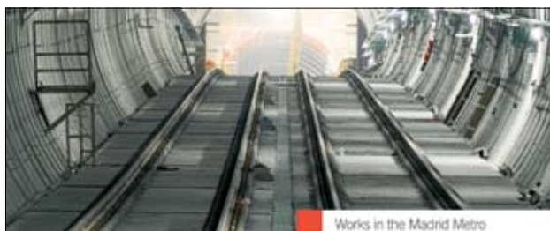
Works in the Madrid Metro
