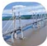
The Second Bridge Spanning the Orinoco River Venezuela
