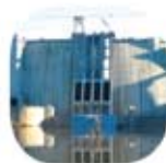
Alqueva's Hydroelectric Development Portugal
