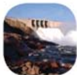
Capanda Hydroelectric Power Plant Angola
