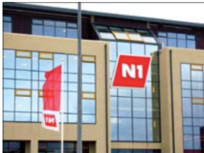
N1's new building.
