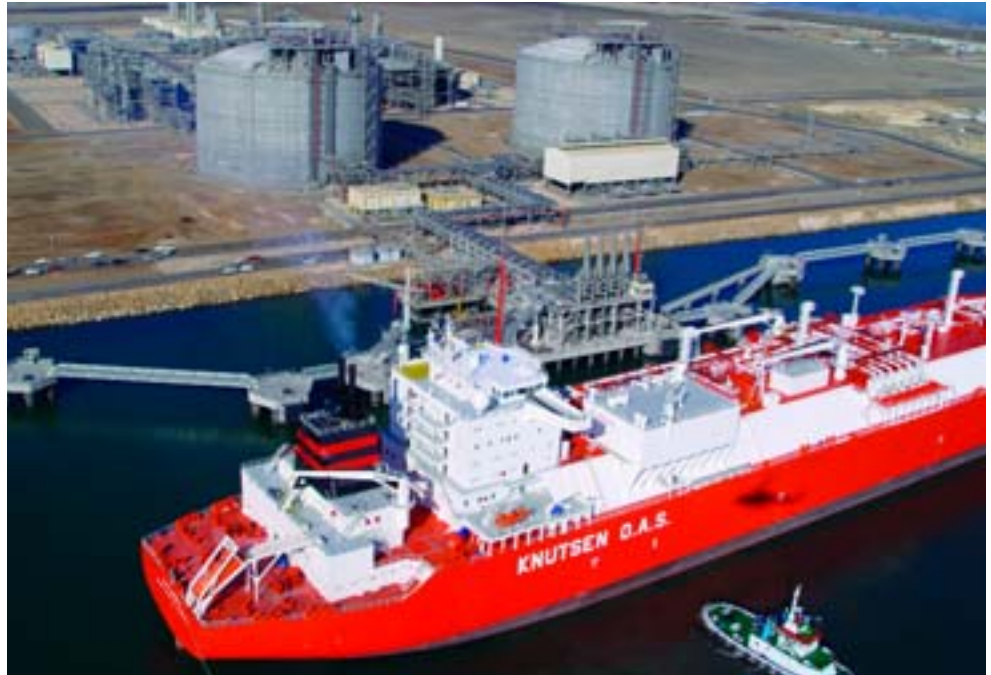
Mubarak 2 Gas & Petrochemical Complex.
