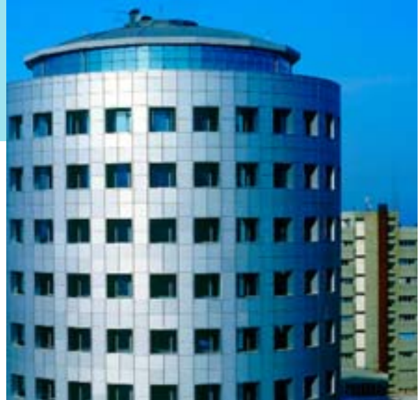
New facilities are being built
