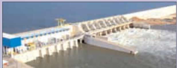
Peixe Angical hydroelectric plant
