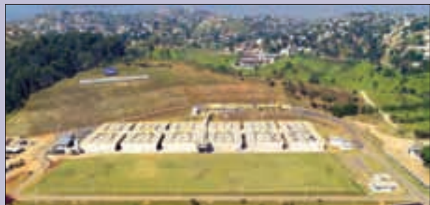
Sewage treatment plant, Belo Horizonte, Capital of Minas Gerais State
