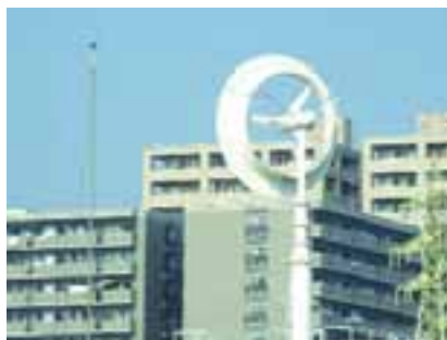
Unlike conventional wind turbines, the wind lens is small and quiet so it can be placed in densely inhabited areas.
