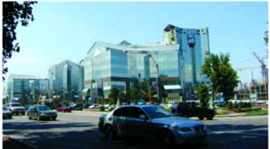
"NurdyTau" business center under construction
