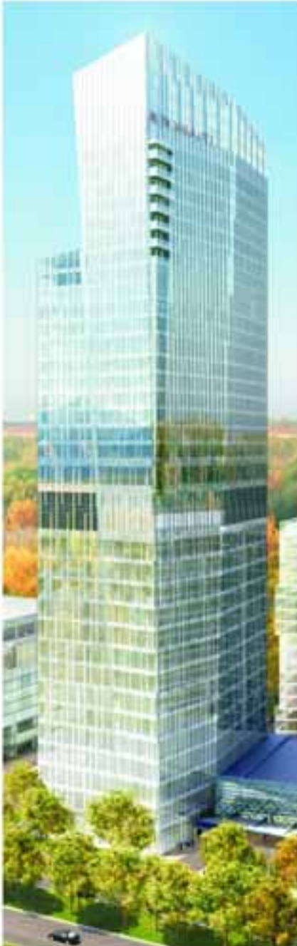
J. W. Marriott building under construction
