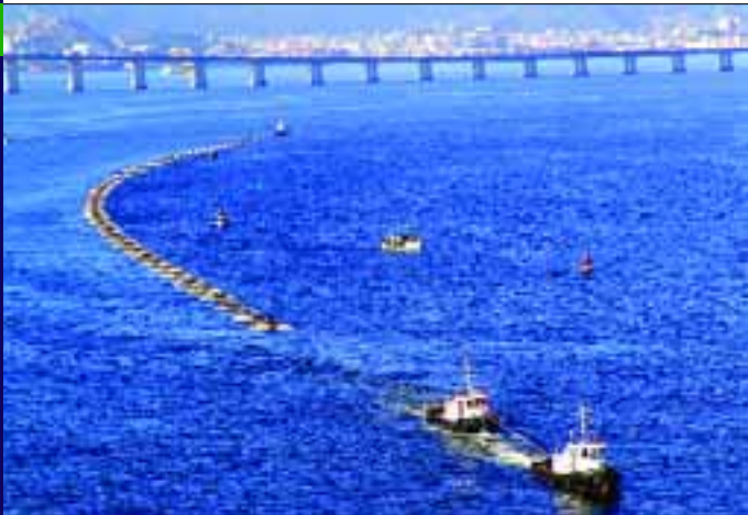
GDK: Constructing and rehabilitating submarine pipelines along the Brazilian coastline www.gdksa.com
