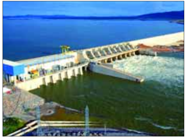
Peixe Angical: adding 452 MW of power to the Brazilian electricity network
