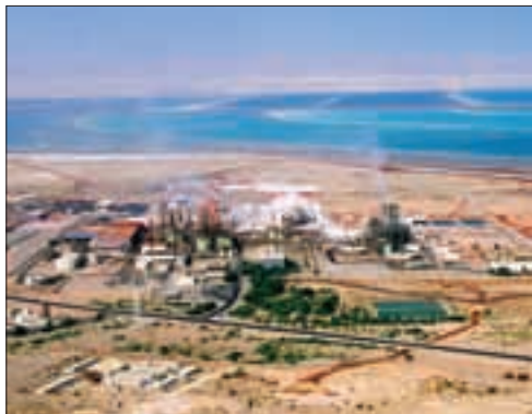
The Potash Refinery complex in Safi
